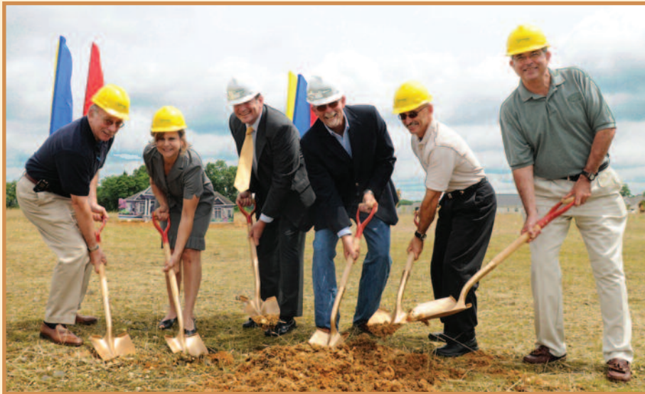
Millville officials joined K. Hovnanian executives in breaking ground on a 7,500-square-foot clubhouse at K. Hovnanian's Four Seasons at Millville. Tossing the first shovelsful of dirt are Dale Finch, Millville commissioner; Jane Jannarone, county freeholder; Duff Henderson, K. Hovnanian community manager; Mayor Tim Shannon; Vice Mayor Joseph Derella; and Earl Sherrick, executive director of the Greater Millville Chamber of Commerce. The community includes 104 single-family homes for adults over 55 years. The clubhouse includes a fitness center, meeting rooms, multipurpose room with kitchen and locker space. Outside the clubhouse will be a swimming pool, a tennis court and a bocce court.
